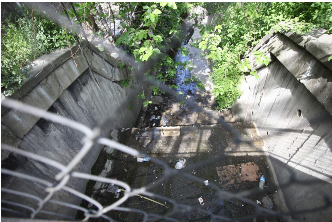
Figure 5.30: Stream under Thresholds (Tavukcu, 2019).
