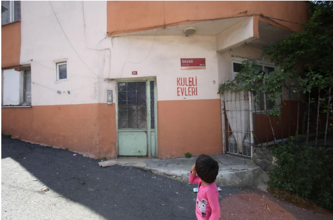
Figure 5.6: The building next to Kuleli Evleri (Tavukcu, 2019).
