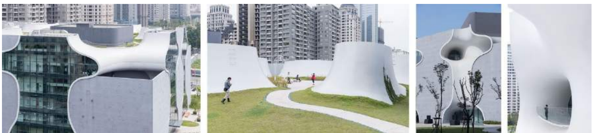
Figure 2.7. (a)(b) The roof garden of the Taichung Metropolitan Opera House. (c)(d) Terraces of the Taichung Metropolitan Opera House (URL-13)
