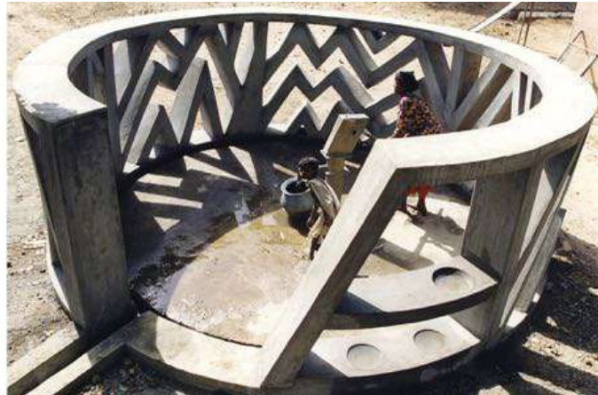
Figure 1 A re-designed water fetching structure at Bandapara, DIAA, India, 2001
