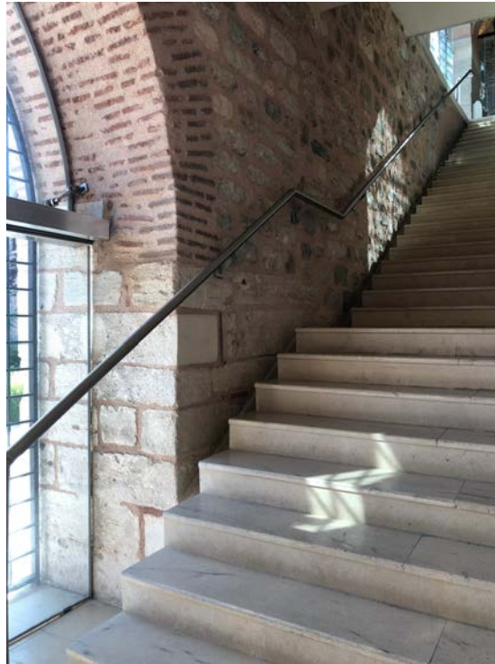
Figure 3.13. Staircase to the second floor
