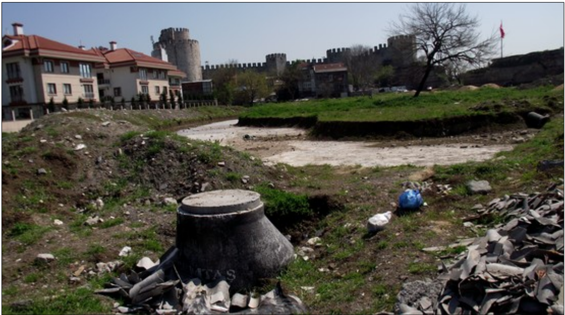
Figure 22: Fertile and green Bostans destroyed and dug up to expand the “Yedikule Residences” urban transformation project
