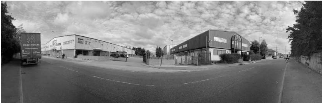
Figure 63: Photo from the road to The Warehouse (located on the right)
