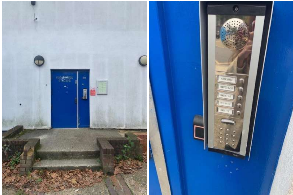
Figure 77: Photos from Sugarhouse Studios entrance
