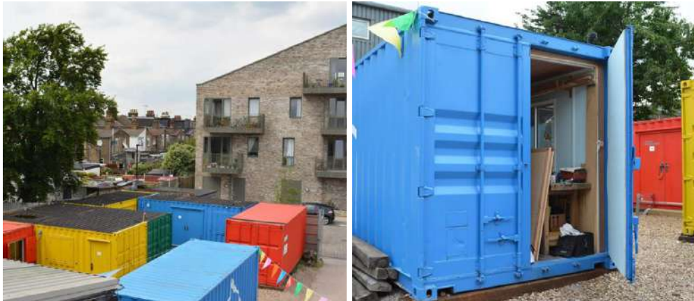
Figure 52: Converted shipping containers
