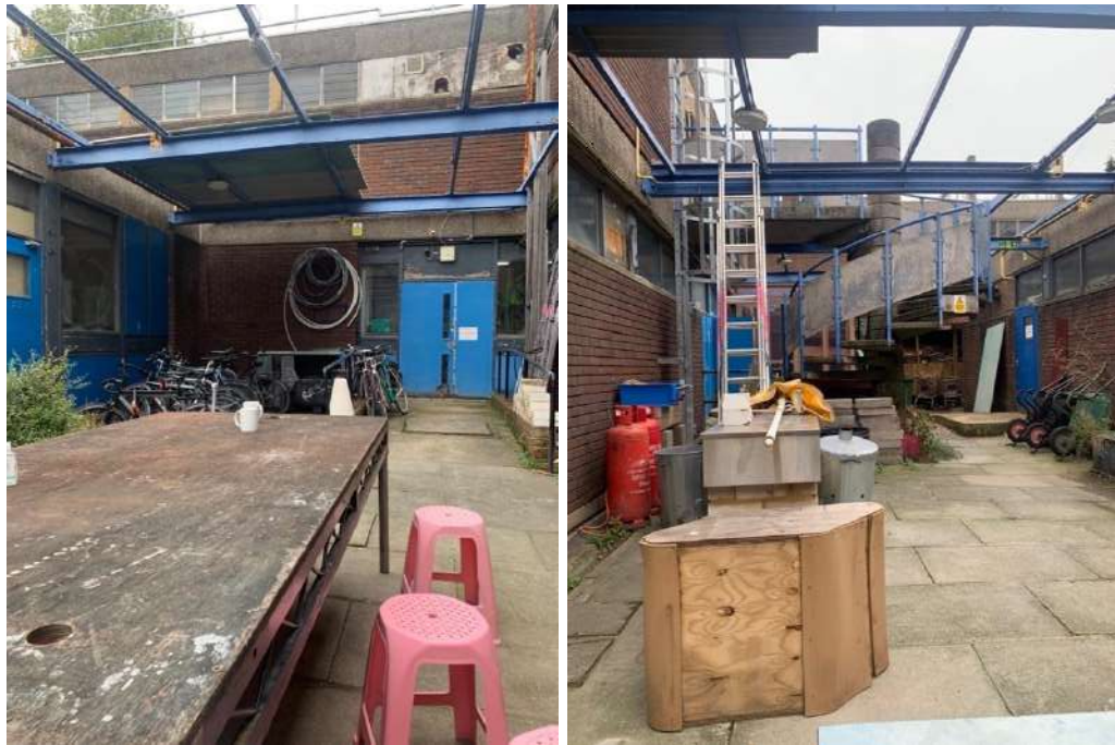
Figure 80: Photos from the courtyard
