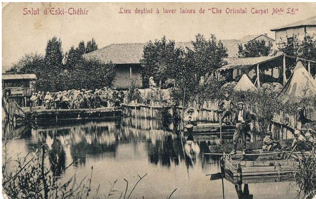
Appendix G-8: OCM's wool washing facilities at Eskişehir.
