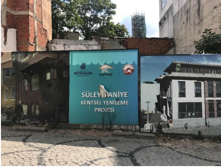
Figures A.1 Information Billboards Surrounding the Renewal and Restoration Project in Süleymaniye District
