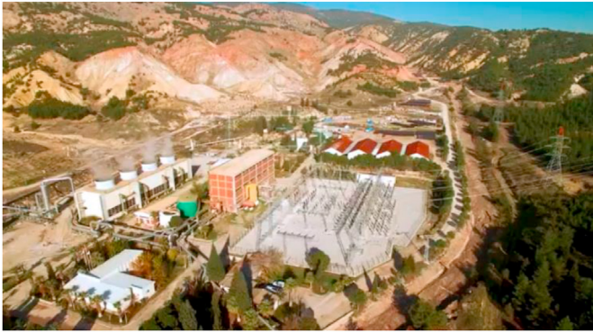
Fig. 7. Kızıldere-I single flash geothermal power plant in Western Anatolia.
