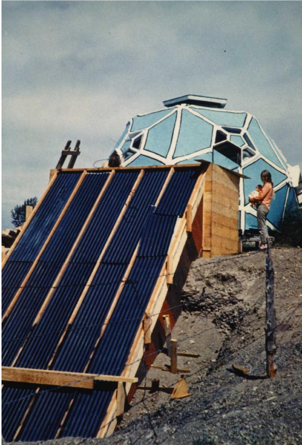
Figure 64. Passive solar collector construction at Drop City, designed by Zomeworks. Photograph by Clark Richert, 1967 (Awan et al 2013).
